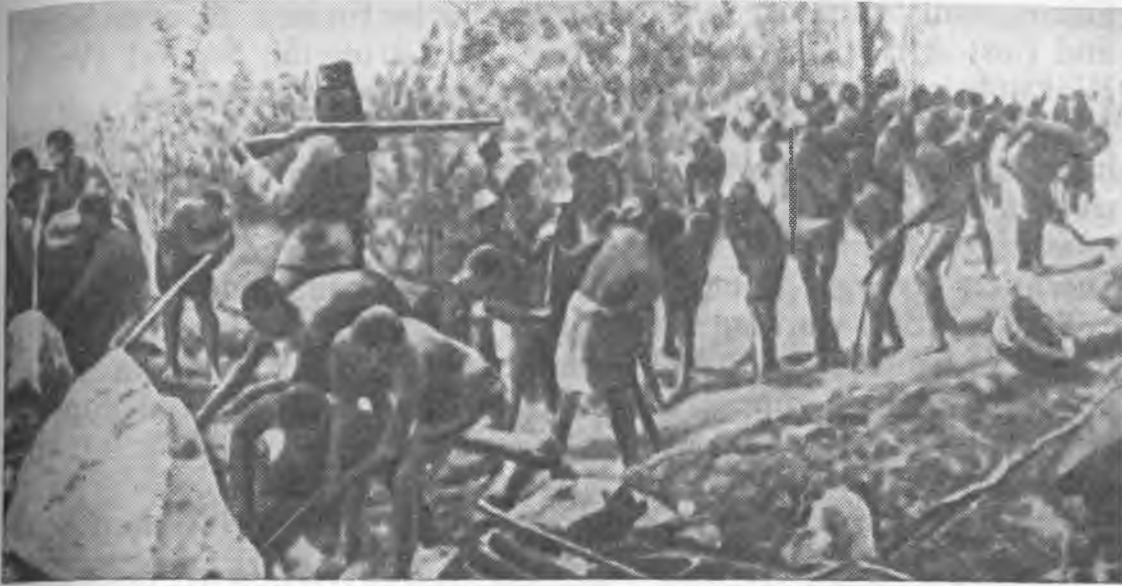
Building a road in the Congo
