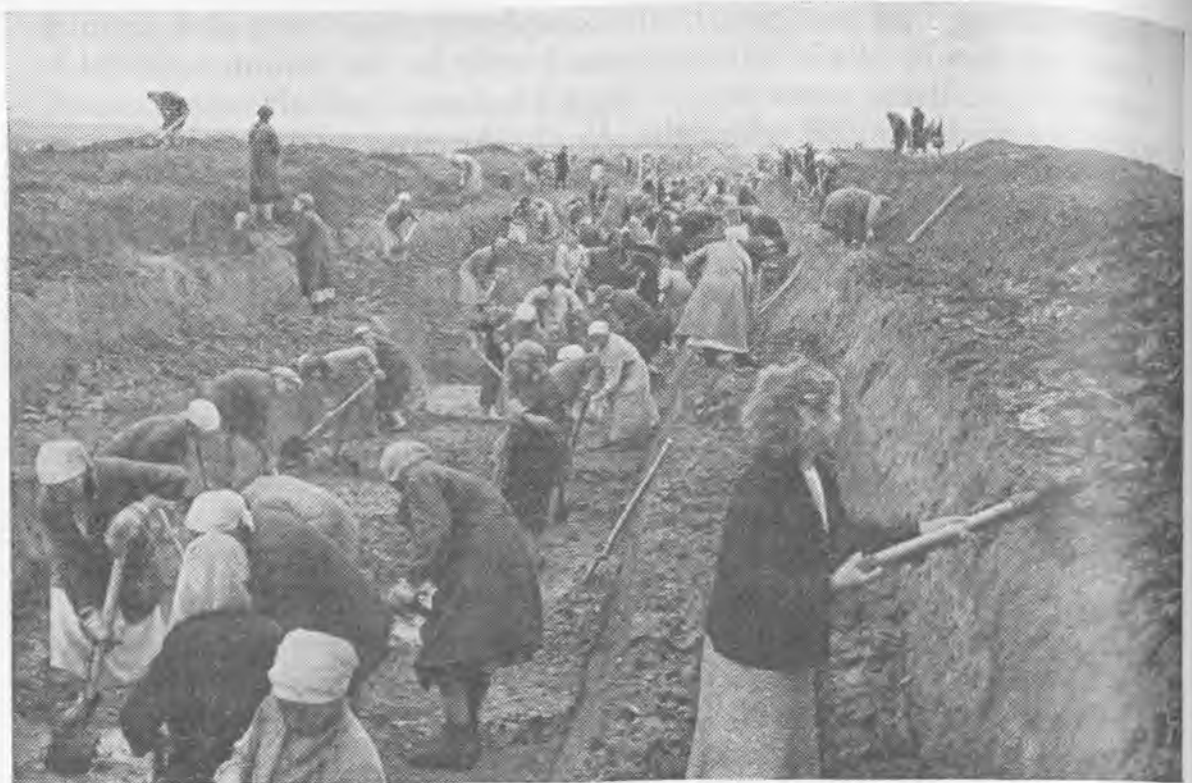
Digging tank ditches in vicinity of Moscow (October 1941)
